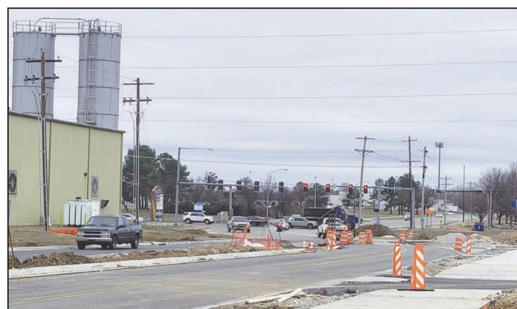
Construction on Water Tower Road as seen from NWACC’s east driveway.
